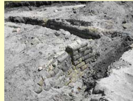
**Trench walls of gun emplacements, lined with sandbags consolidated with cement and metal rods.**
